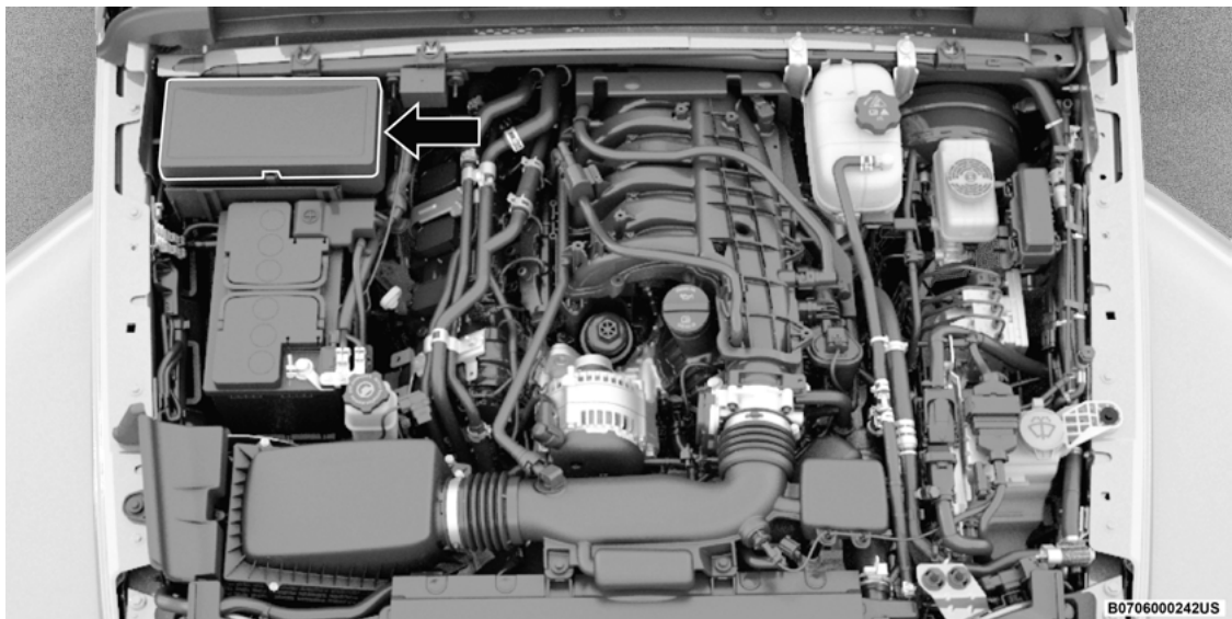
Power Distribution Center Location
