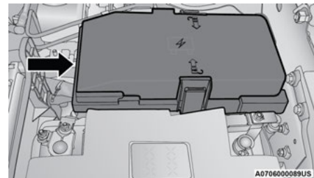
Power Distribution Center
