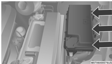
Totally Integrated Power Module
