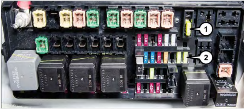
Power Outlet Fuses
