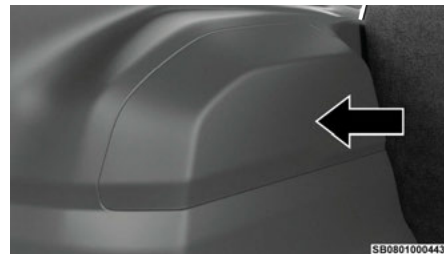
Rear Power Distribution Center Location
